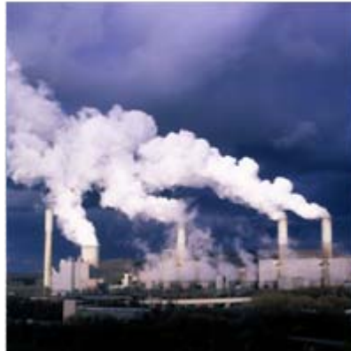
Power station 1,000 MW
